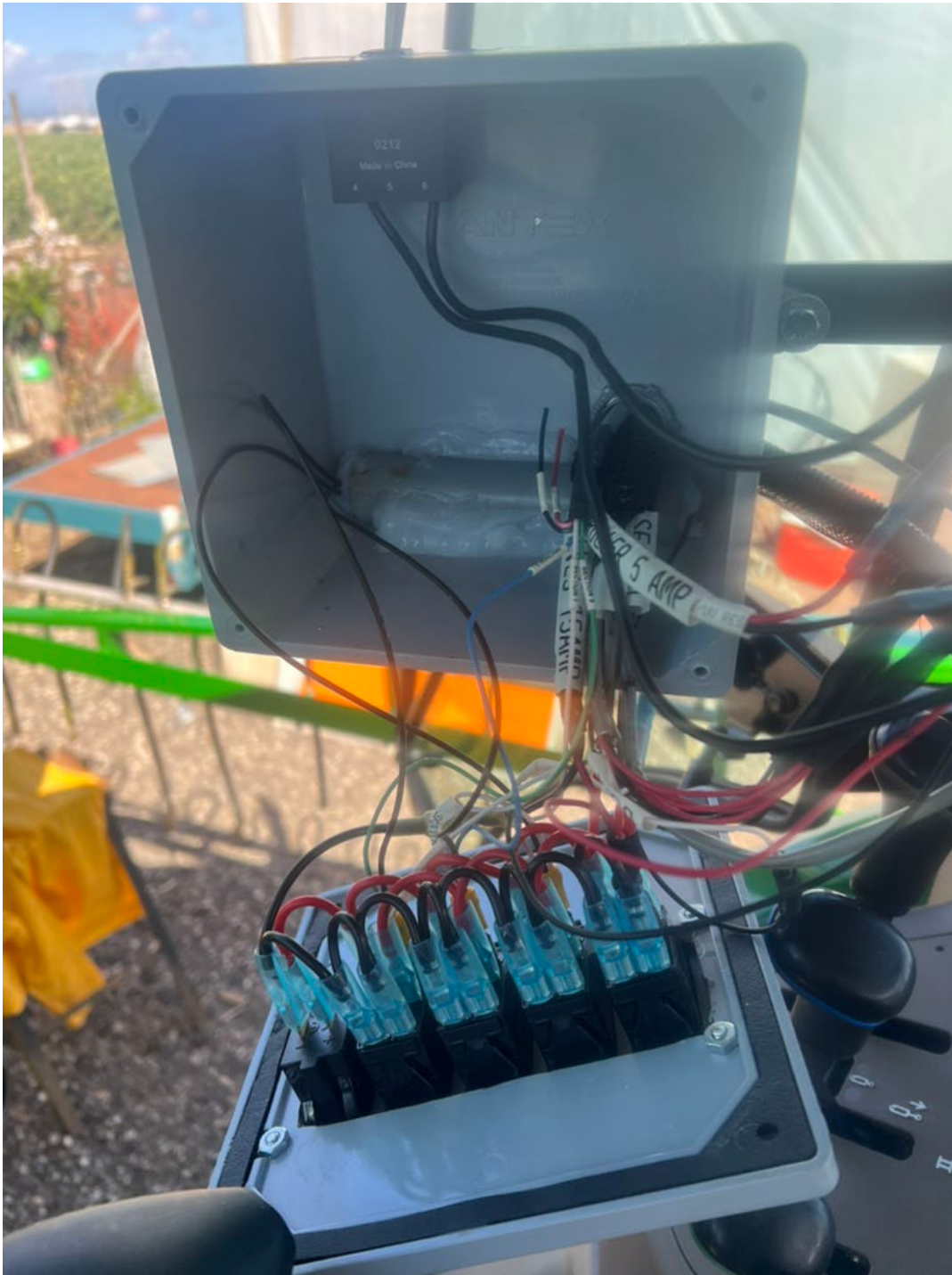
Custom built switchbox attaching BOOM SENSE at the back of switches
